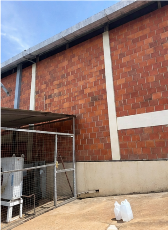
EXISTING PACKHOUSE (RAISED VERANDA TO BE DEMOLISHED)
