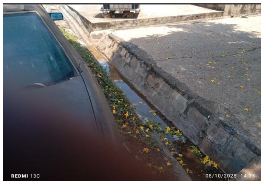
Open drainage channels at the Kenya Border post
