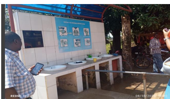
A well-built handwashing facility at the Uganda border post.
