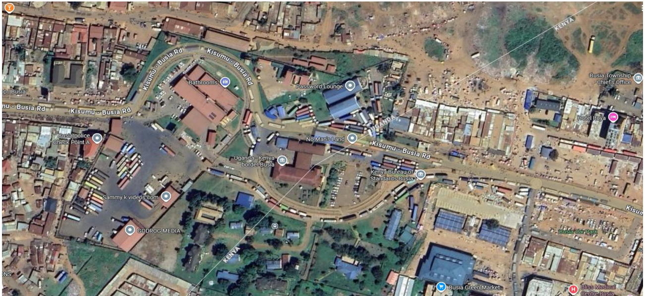
Figure 3: Aerial Image of Busia OSBP
