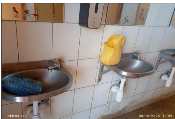
Public sanitary facilities at the Uganda OSBP
