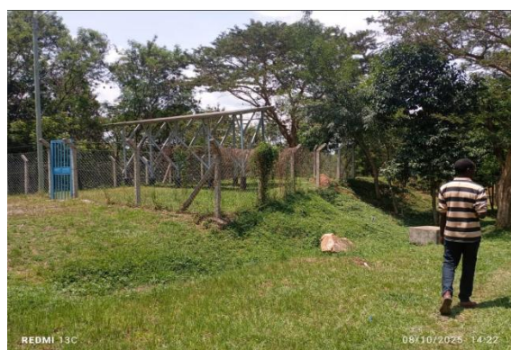
Existing solar system for water pumping
