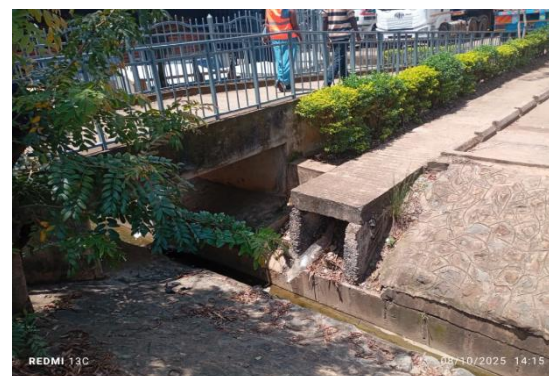
Drainage channels at the Kenya OSBP
