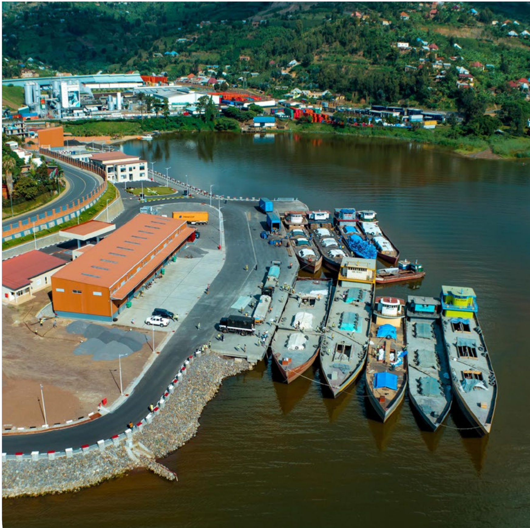
Rubavu Port, Lake Kivu, Rwanda. Officially launched in December 2024, the two hectare port was developed under Rwanda's National Strategy for Transformation backed by partners including the UK (via TMA) and Netherlands-backed Invest International. Designed to handle up to 700,000 tonnes of cargo and 2.7 million passengers a year, it is meant to shift trade onto the lake, cut transport costs and tighten links with Rwanda's trade neighbours while also supporting local jobs through port operations. Rubavu is the first of four Lake Kivu ports that will be developed by 2029, and a test of whether modern infrastructure can be both efficient and sustainable.
