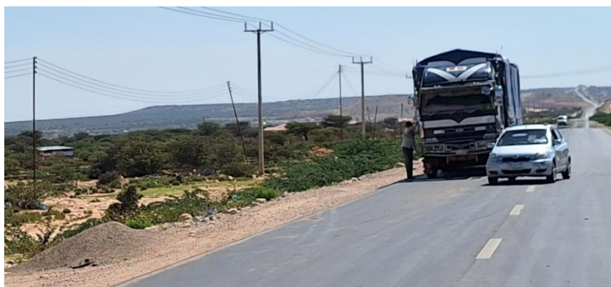
Figure 20 :Example of a lack of paved stopping points along Hargeisa Bypass
