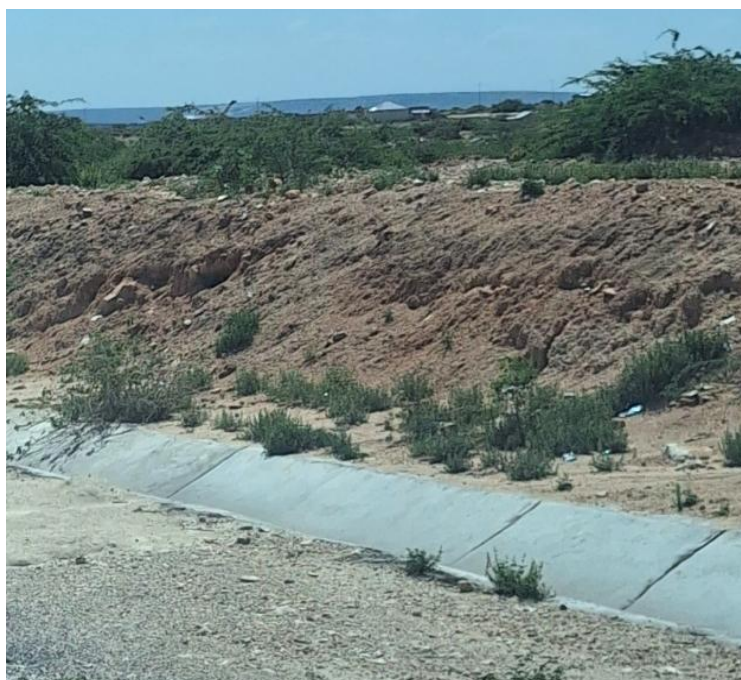
Figure 22 Example of drainage along Hargeisa Bypass, Somaliland
