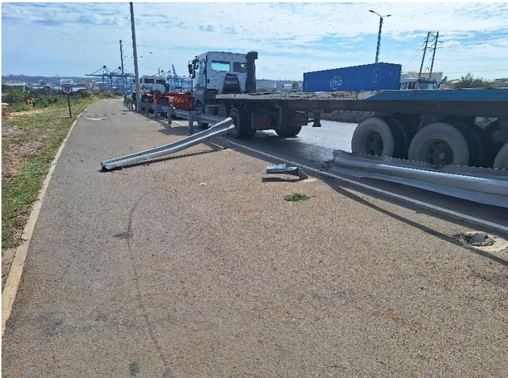
Figure 21 Example of road barrier damage at Kipevu Road, Mombasa
