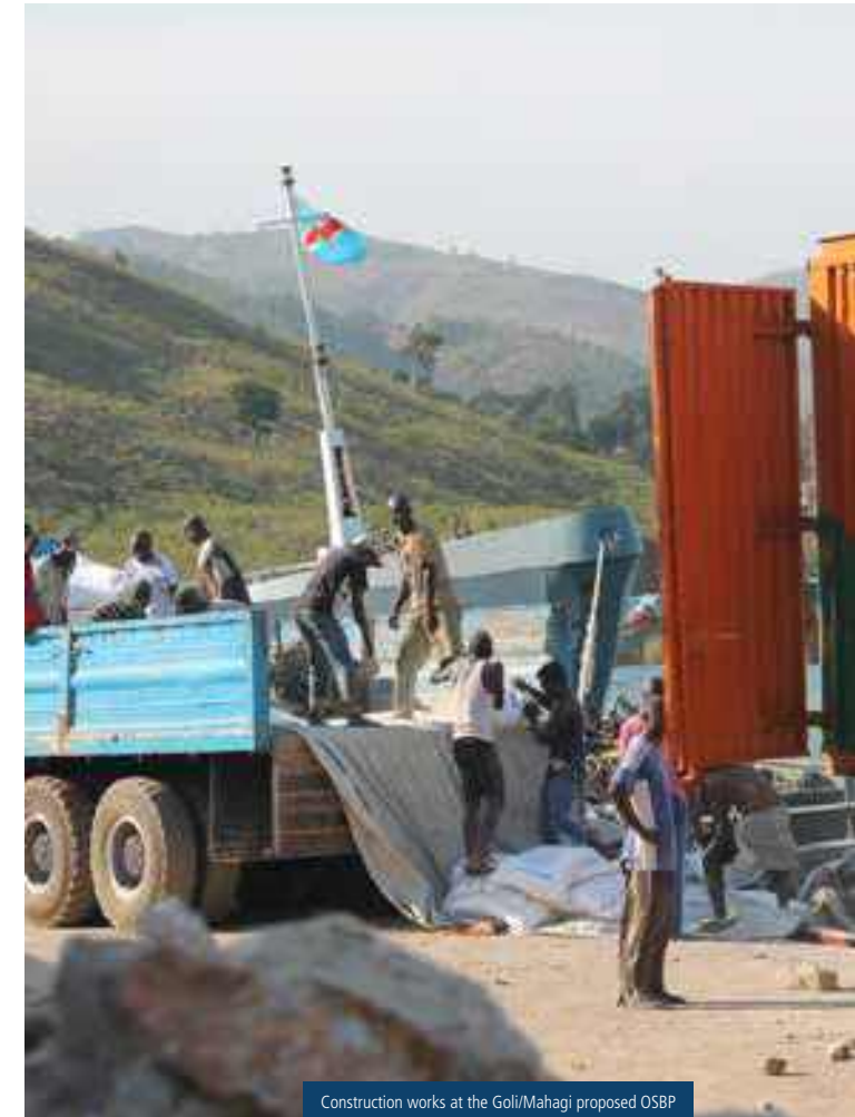
Construction works at the Goli/Mahagi proposed OSBP
