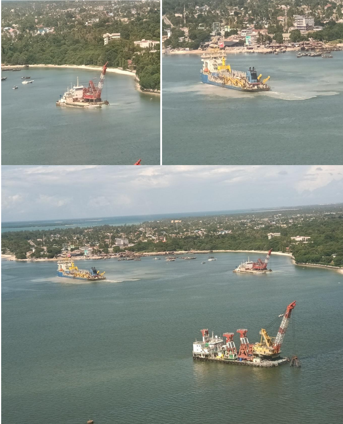
Dredging works in progress
