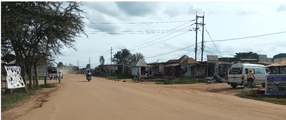
Feeder and/or access roads on the main road to Mutukula OSBP within the control zone on the Tanzanian side
