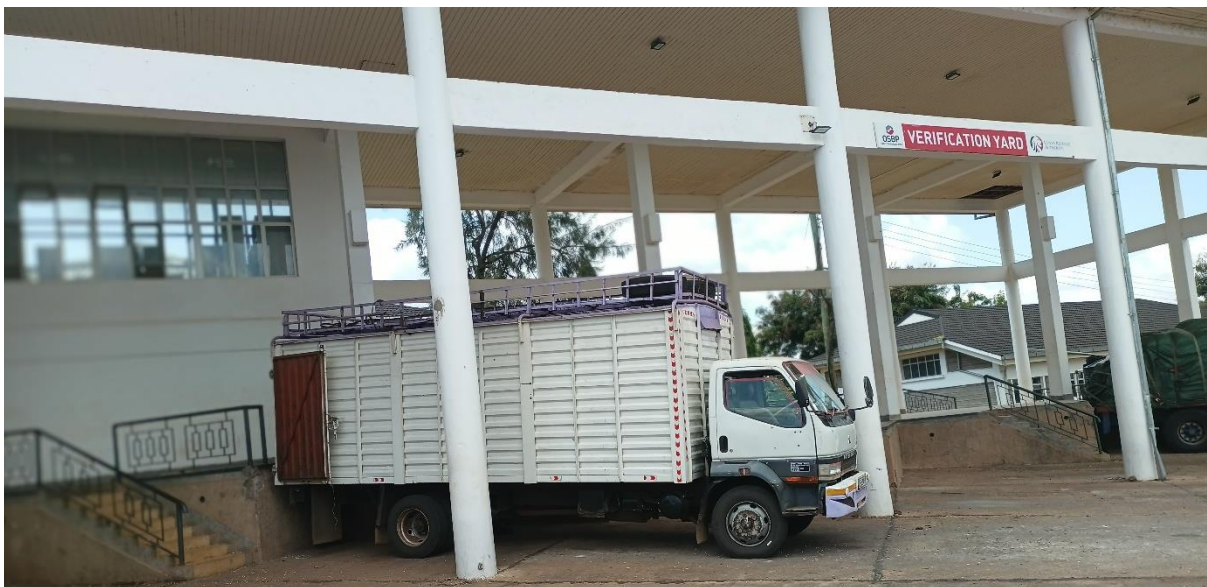
Trucks verification bay at Taveta OSBP
