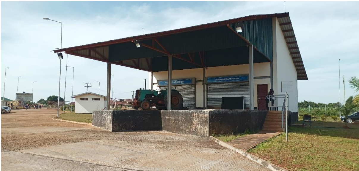
Truck verification yard at Kabanga OSBP
