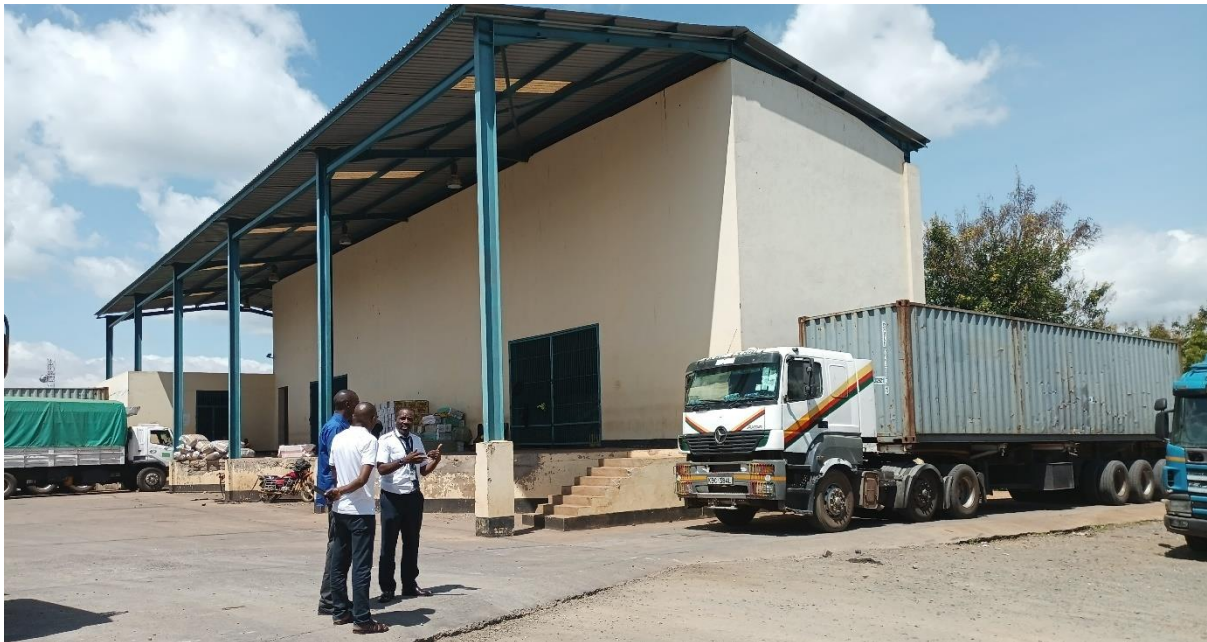
Trucks verification bay at Holili OSBP
