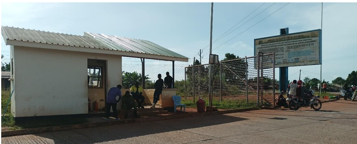
Typical guard house used by several border officers for control of exit protocols at Kabanga OSBP
